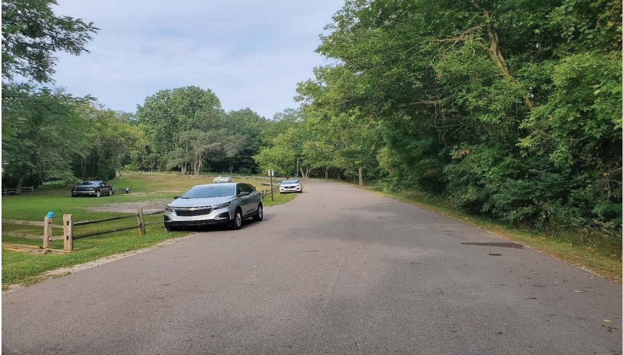
ROADWAY LOOKING WEST, NORTH OF DAM CONTROL STRUCTURE
