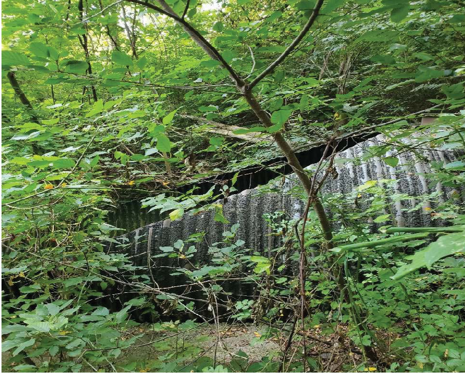
DOWNSTREAM CORRUGATED METAL PIPE OUTFLOW DISCHARGE
