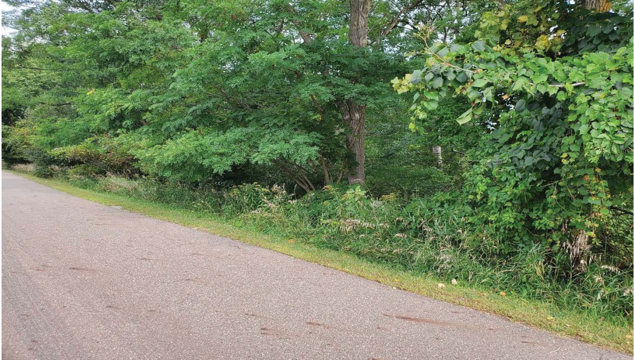
NORTH OF ROADWAY EMBANKMENT, WITH TYPICAL TREE AND BRUSH GROWTH THROUGHOUT
