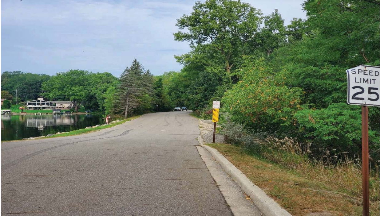
EMERGENCY SPILLWAY LOOKING WEST
