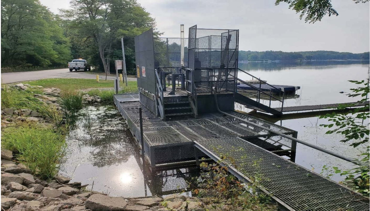
LOOKING EAST TOWARDS DAM CONTROL STRUCTURE
