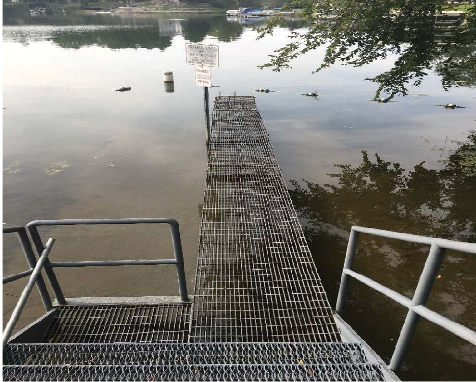
LOOKING SOUTH TOWARD LAKE FROM DAM CONTROL STRUCTURE
