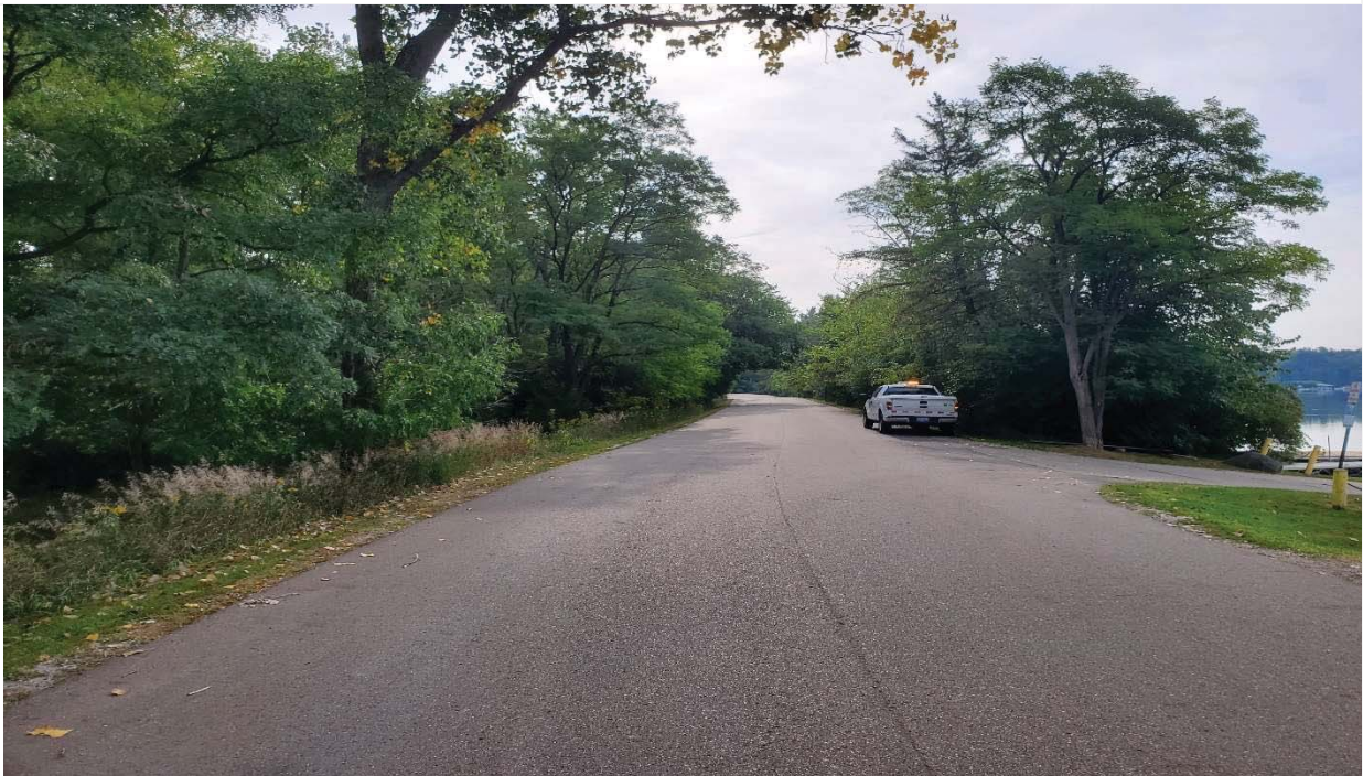
ROADWAY LOOKING EAST, NORTH OF DAM CONTROL STRUCTURE
