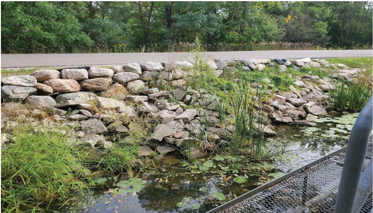
RIPRAP NORTH OF DAM CONTROL STRUCTURE, ALONG EMBANKMENT
