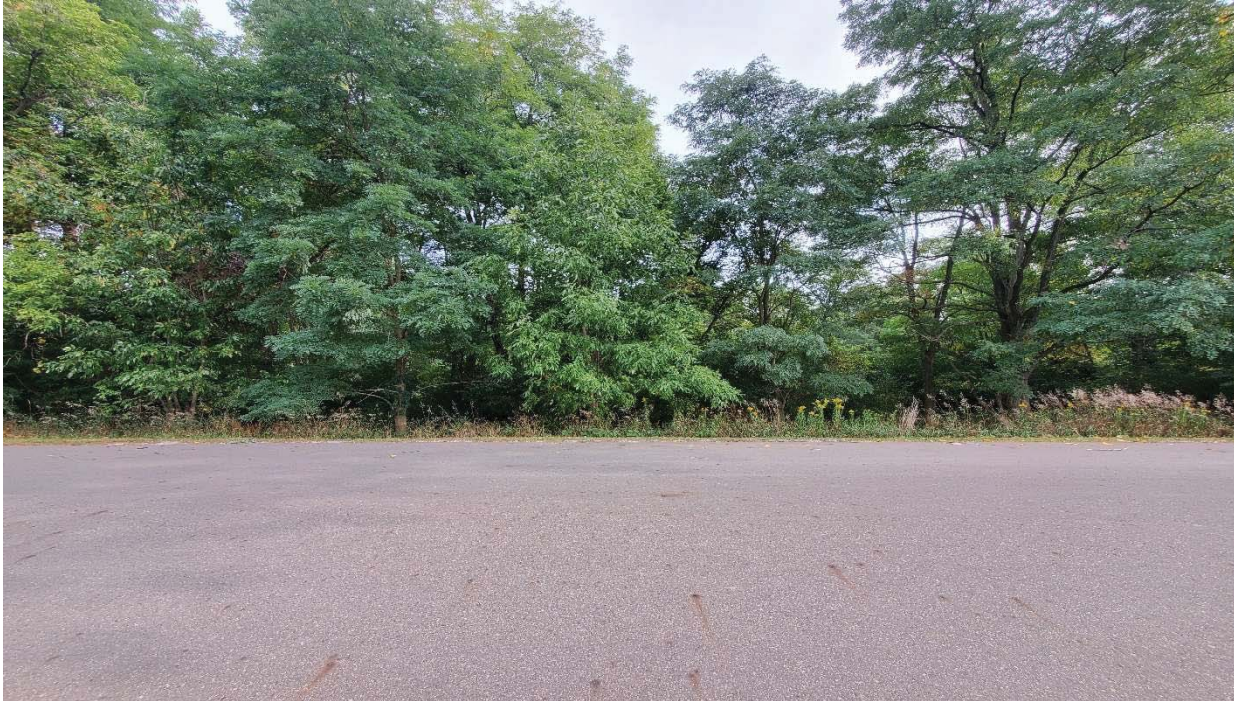
ROADWAY NORTH OF DAM CONTROL STRUCTURE LOOKING NORTH TOWARDS NORTH EMBANKMENT
