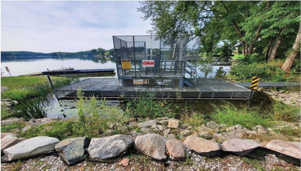
LOOKING SOUTH TOWARDS DAM CONTROL STRUCTURE
