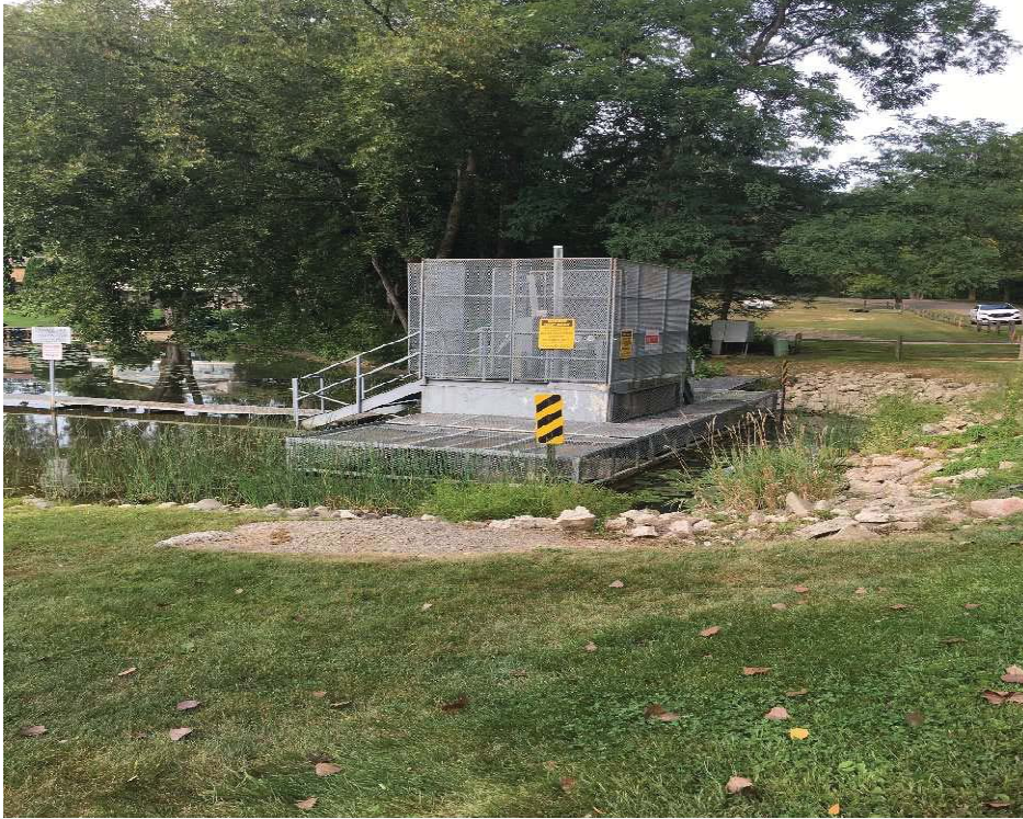
LOOKING WEST TOWARDS DAM CONTROL STRUCTURE
