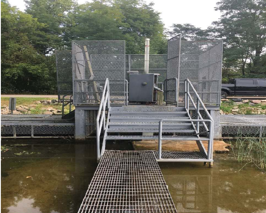
LOOKING NORTH TOWARD DAM CONTROL STRUCTURE
