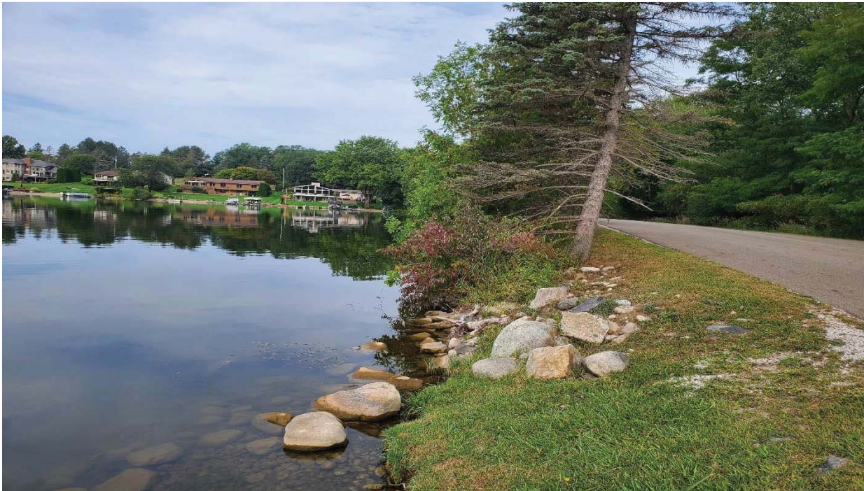
TYPICAL SOUTH EMBANKMENT OF LAKE SHANNON NEAR EMERGENCY SPILLWAY
