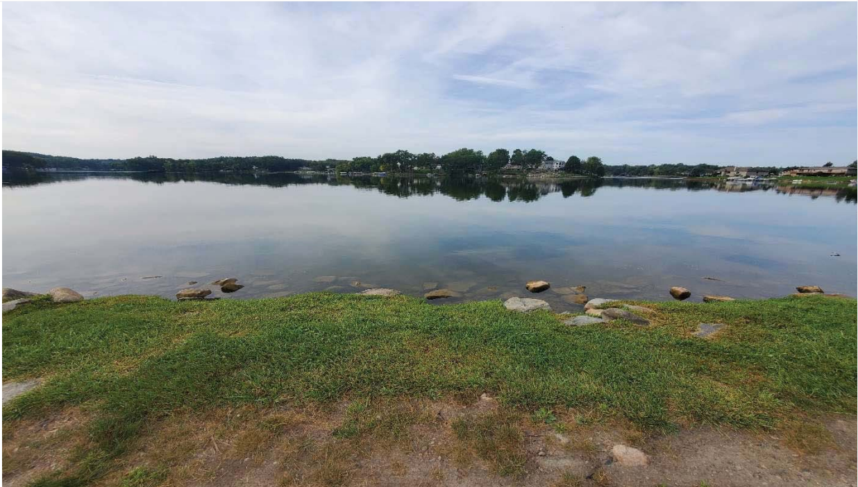
SOUTH EMBANKMENT OF EMERGENCY SPILLWAY LOOKING SOUTH TOWARD LAKE
