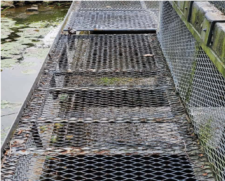
TYPICAL GRATING AND SUPPORT SYSTEM @ CONTROL STRUCTURE
