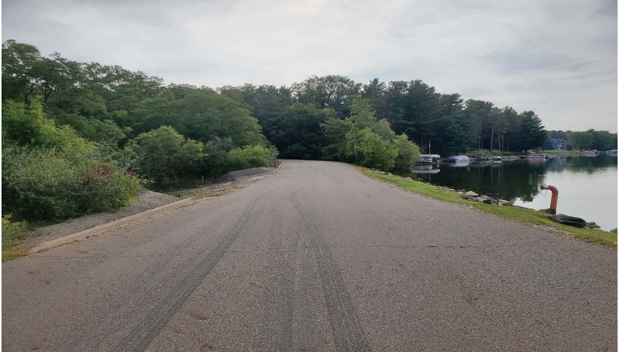
EMERGENCY SPILLWAY LOOKING EAST
